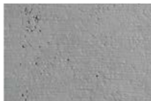
Coarse concrete technique
